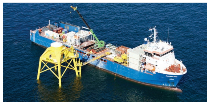
Grouting Telescopic crane
