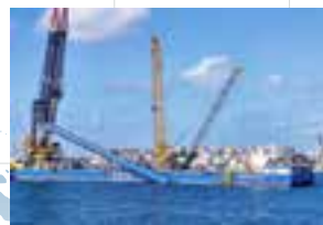
20 Port Said [Egypt] Pile installation for floating dry dock Page 53
