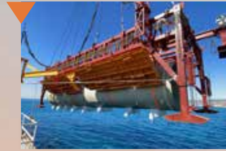
GRP pipe installation with specially engineered hoisting frame.
