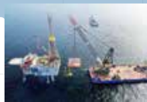
12 Trinidad & Tobago DeNovo Energy Topside installation Page 31
