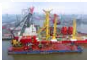
5 Rotterdam [The Neth.] Ceona Amazon Installation works Page 19
