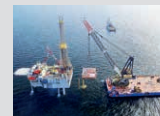
Trinidad & Tobago DeNovo Energy Topside installation
