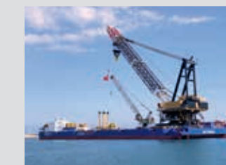
Akkuyu [Turkey] Nuclear powerplant Subsea installation
