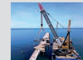
Sagunto [Spain] Removal of jetty infrastructure
