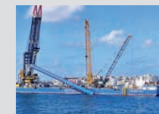
Port Said [Egypt] Pile installation for floating dry dock
